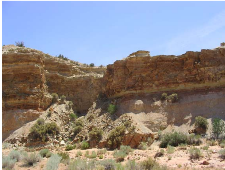
Photo 7. Photo taken looking south. Fault graben located within the Carmel Formation. Caused by gypsum withdraw.
